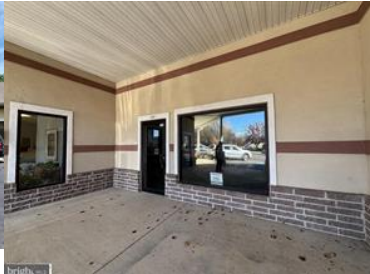
Exterior facade, door, window to #104
